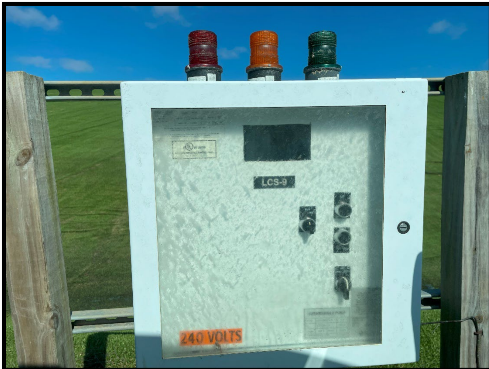
Photograph 2: View of missing display in LCS-9 panel.
