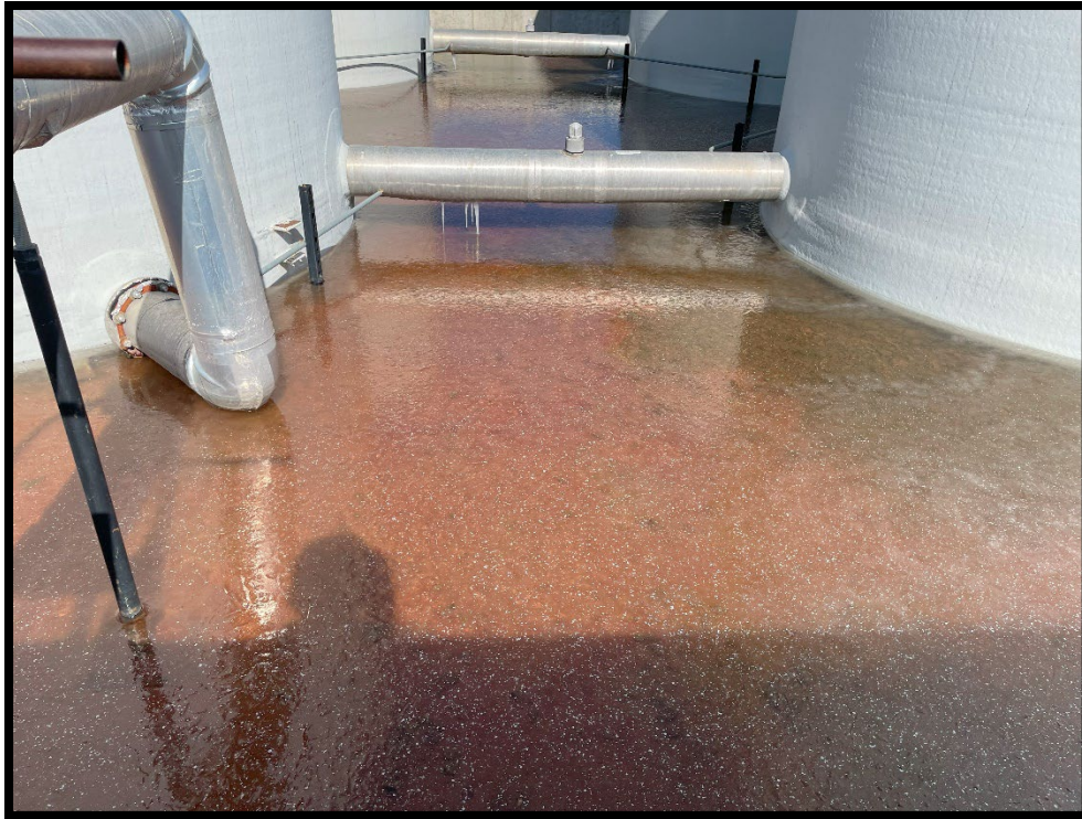
Photograph 1: Secondary containment frozen solid.
