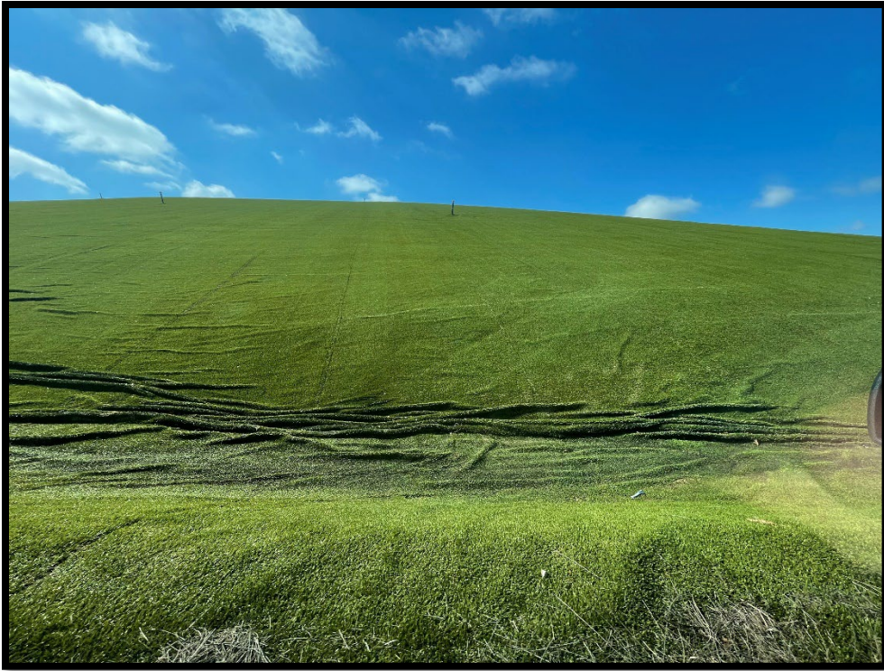
Photograph 3: View of rills near LCS-1.
